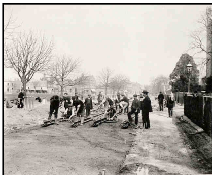
Laying tram tracks on Hampton Road on 18th March 1902. The tower of Holy Trinity church can just be made out on the right
