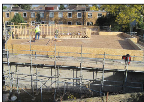
The Contact Centre under construction, seen from Pope's Avenue
