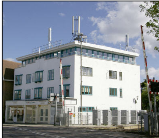
Three of the five masts on Rochester House
