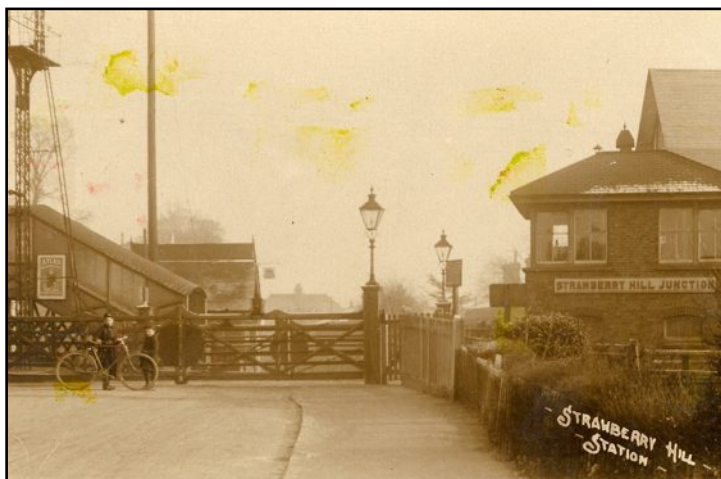
The level crossing in the early 20th century. The structure of the footbridge can be seen.
